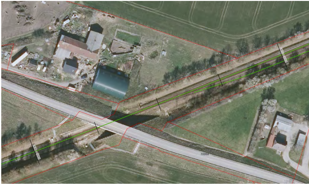
Figur 5: Sporskifte St. 230.870 - St. 230.910, (km 156.825)
