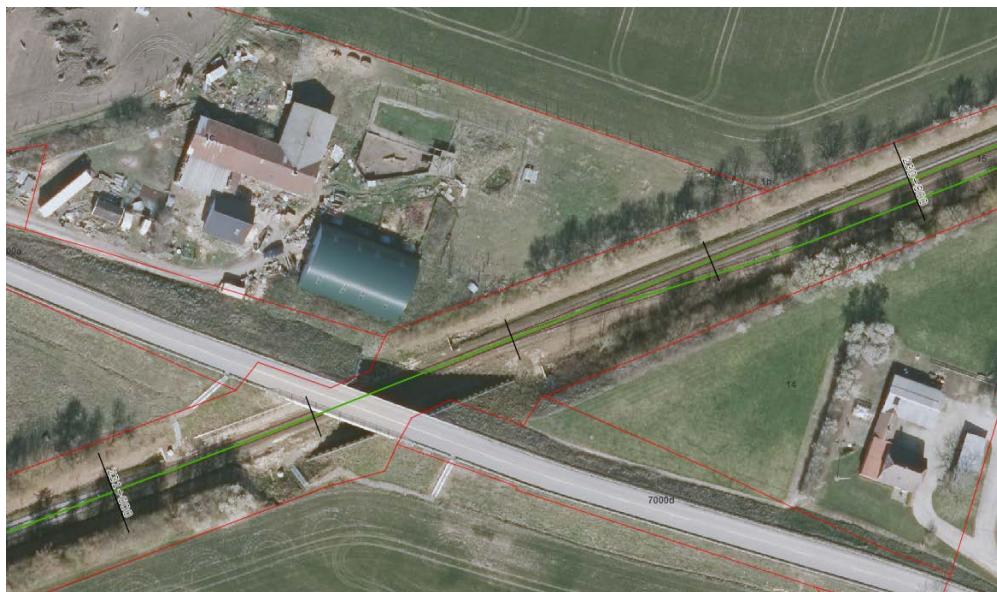
Figur 5: Sporskifte St. 230.870 - St. 230.910, (km 156.825)
