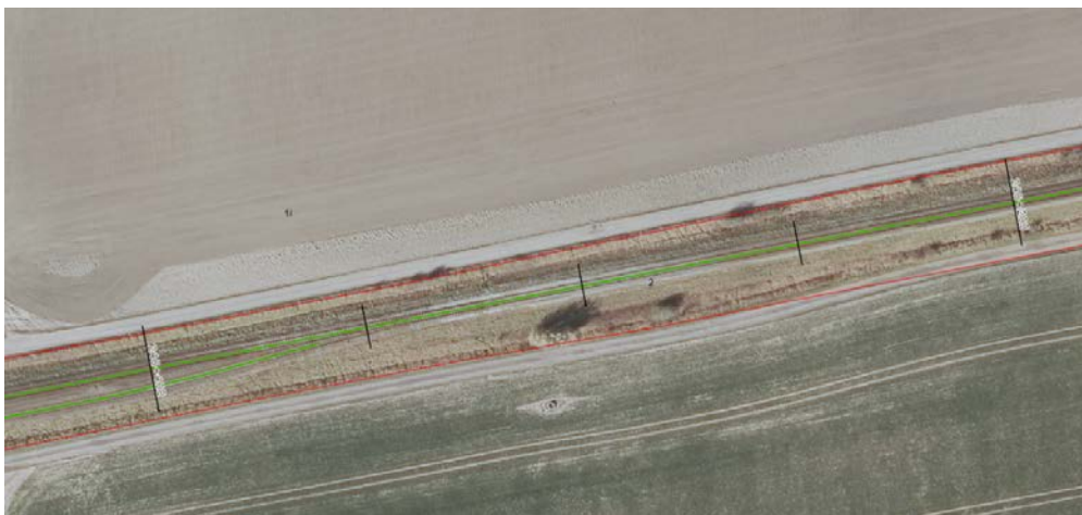
Figur 8: Sporskifte St. 246.320 - St. 246.370, (km172.300)
