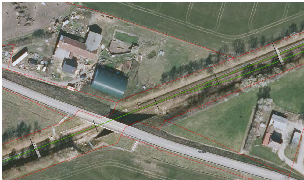
Figur 5: Sporskifte St. 230.870 - St. 230.910, (km 156.825)
