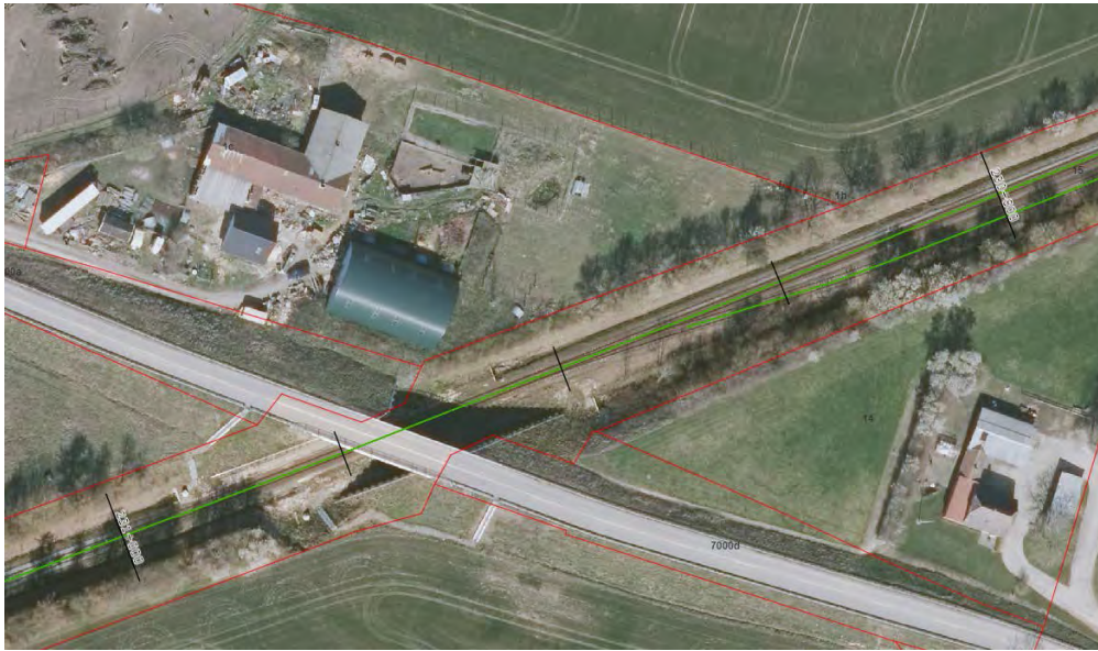
Figur 5: Sporskifte St. 230.870 - St. 230.910, (km 156.825)
